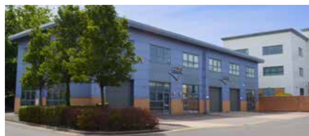
Corporate Headquarters & Warehouse Facilities
